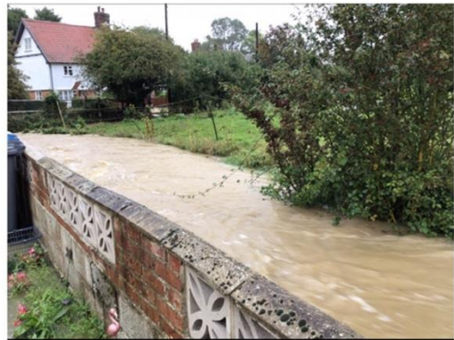
L: View from the gull towards Bridge Street
