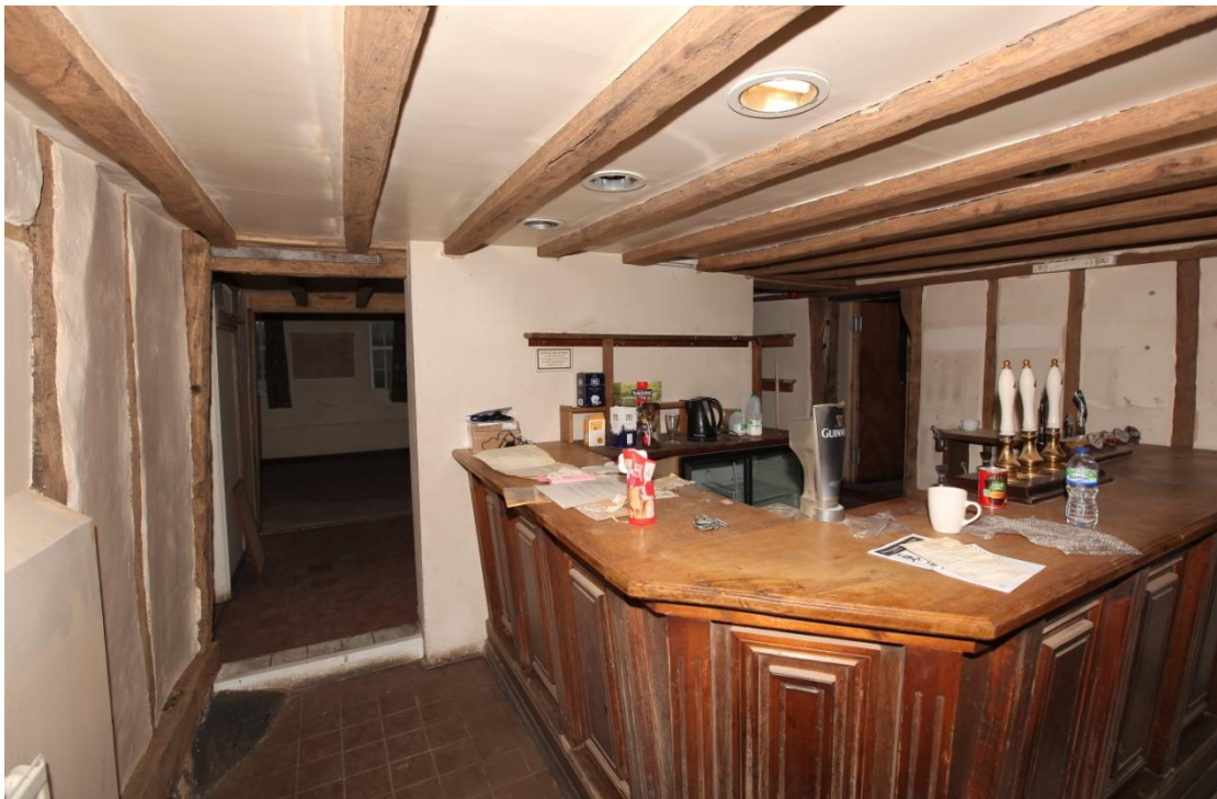
Illus. 9. The service bay of the 16 th century house (A1), seen from the north. The ceiling joists may be original but have been re-set and are now secured by late-20 th century wire nails. This room was originally divided into a pair of store rooms with an axial partition and a stair to the rear (right). The solid wall in the centre of this image appears to consist only of late-20 th century masonry but occupies the position of the original Tudor gable.
