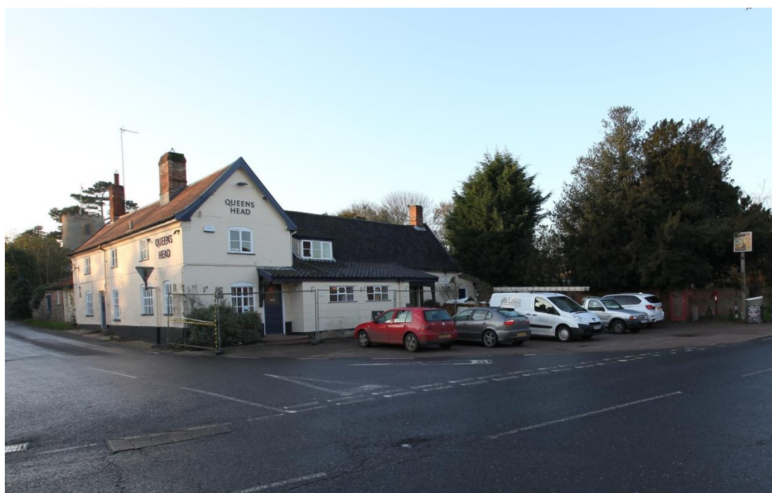
Illus. 1. The inn from the crossroads to the south-east showing the narrow 18 th century wing (B) to the left of the lower 16 th century range (A). The front (eastern) lean-to has been extended to the north since the 1920s (figures 6 & 7), removing the tall chimney, and the easternmost entrance of the cross-wing has moved to its gable.
