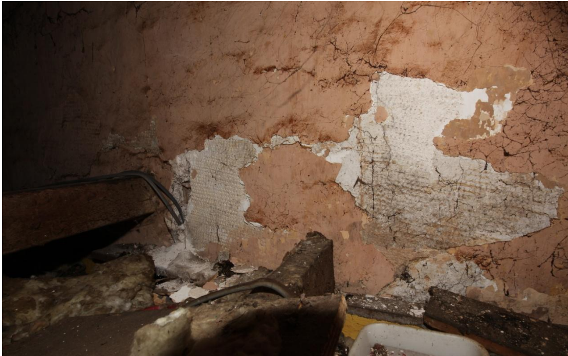
Illus. 16. A detail of the original external plaster above the modern kitchen, as shown to the right in illus. 15 above. The ‘basket-weave’ pargeting to the lime plaster illustrates the wall’s original appearance (contrasting with the brickwork of the western facade), but the red ochre pigment is a 19 th century addition that illustrates an authentic version of ‘Suffolk Pink’.
