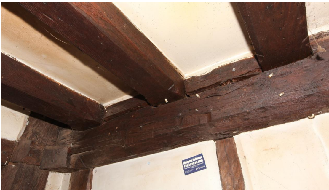
Illus. 15. A detail of the high-quality 16 th century ceiling joists in the north-eastern corner of the rear room (B3). Note the chamfer stop to the left of the principal joist, which is matched at its opposite (southern) end and indicates the ceiling was designed for a building of the same unusually narrow width (with just 12 ft or 3.6 m between its posts). The timber is lodged alongside the post of the northern wall on the left and is not integral to the frame.
