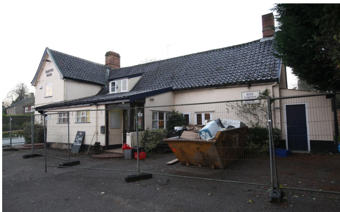
Illus. 2. The 1.5 storied 16 th century house with its glazed black pantiles and enlarged lean-to addition. The original timber-framed structure (A) terminated beneath the left-hand mullion of the dormer window but was extended in the late-18 th century to meet the new cross-wing (B). The right-hand section of the facade has been rebuilt in brick.
