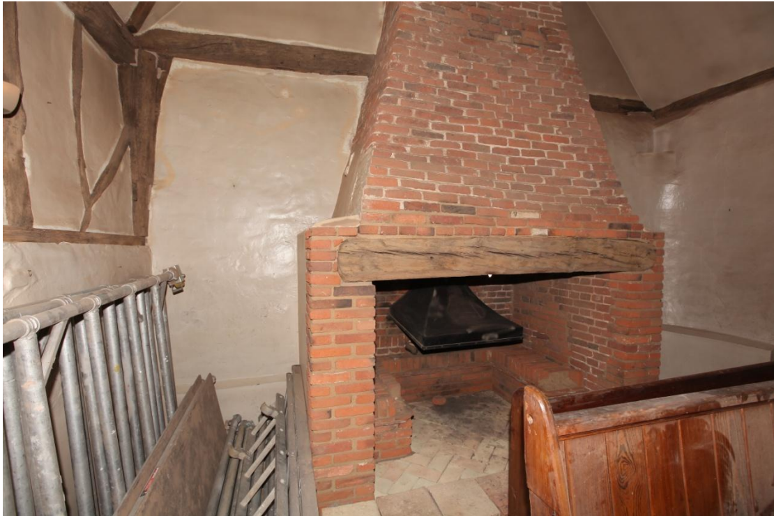
Illus. 7. The 17 th century chimney at the northern end of the 16 th century hall (A2). The brick piers were rebuilt in the late-20 th century and the timber lintel replaced. This fireplace may have operated in conjunction with the original ceiling, but may relate to the subsequent conversion of the hall into a bake-house or brew-house. The depth of the fireplace and the curved brickwork on the right suggests it was attached to a bread oven or copper.
