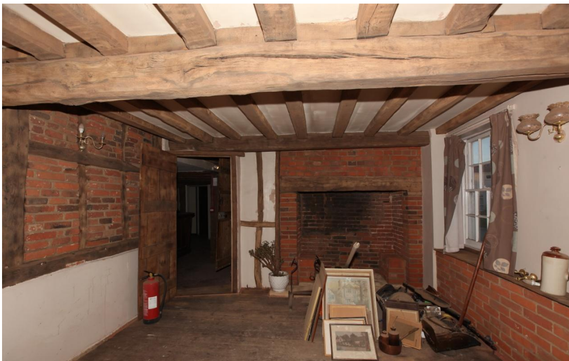
Illus. 13. The central room of the 18 th century wing (B2), seen from the west. The fireplace was largely rebuilt in the late-20 th century but retains some 18 th century brickwork. The timber-framed wall on the left consists entirely of re-used timber, and the high-quality chamfered ceiling joists, which date from the 16 th century, are supported by roughly hewn principal joists of much later date.
