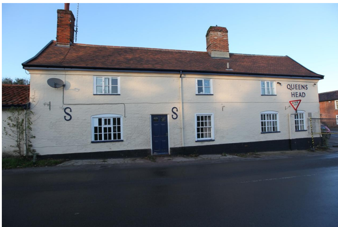
Illus. 3. The brick and tiled southern elevation of the narrow late-18 th century wing. The present door was formerly wider (its original jamb is visible in the brickwork to its right), and the narrow window on the extreme right was initially a second entrance with closers (quarter-bricks) descending to the ground (figure 6).
