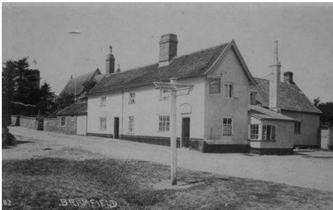
Figure 6. A postcard of the inn from the south-east taken in circa 1920. The southern elevation preserves its two original entrance doors but the present door in the eastern gable of the 18 th century wing is conspicuous by its absence. Note the precariously tall chimney heating the eastern lean-to extension, which may have been the shoemaker's shop, necessary to clear the ridge of the nearby roof.
