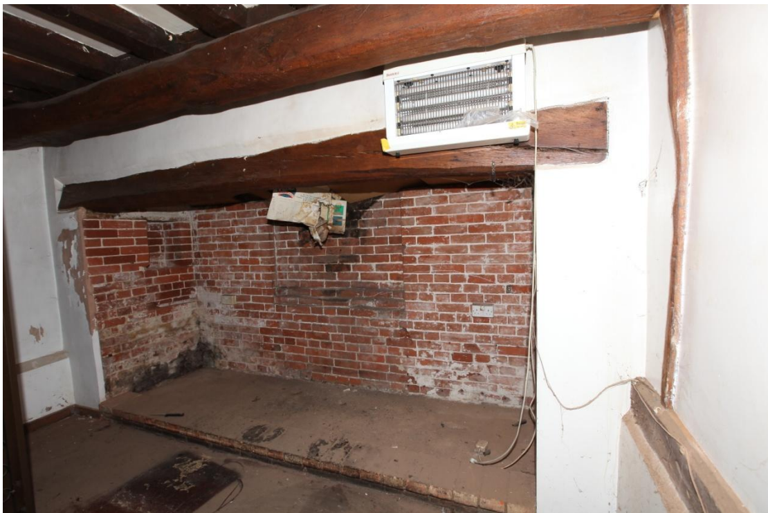
Illus. 17. The imposing original fireplace on the rear (western) gable of the 18 th century wing which served the inn’s small kitchen. This kitchen was entered from the yard on the right and was not connected internally to the rest of the building. The crudely hewn principal joist above the chimney lintel supports the opposite ends of the Tudor common joists shown in illus. 15.
