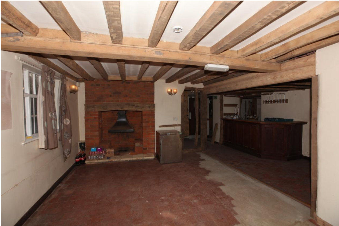
Illus. 12. The front (eastern) room of the 18 th century wing (B1) with the wall marking the original southern gable of the Tudor house adjoining the bar to the right. The plain, re-used ceiling joists here were formerly concealed by plaster, and the fireplace is a 20 th century reconstruction.
