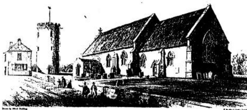
BRAMFIELD CHURCH, FROM THE S. E.
